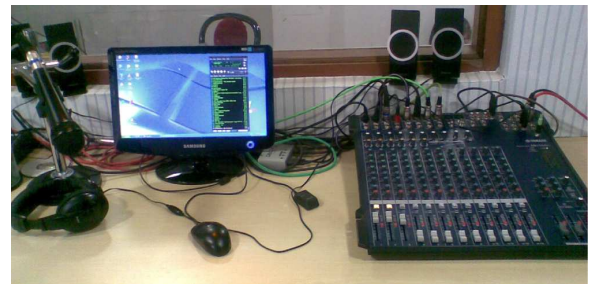
Figure 9: Complexity of mixer settings and cabling at Radio Bundelkhand
